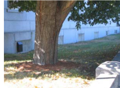
Basement windows allow for potential of additional rentable space on the lower level
