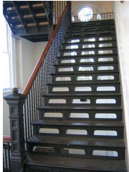
South Stair at Superior Court
