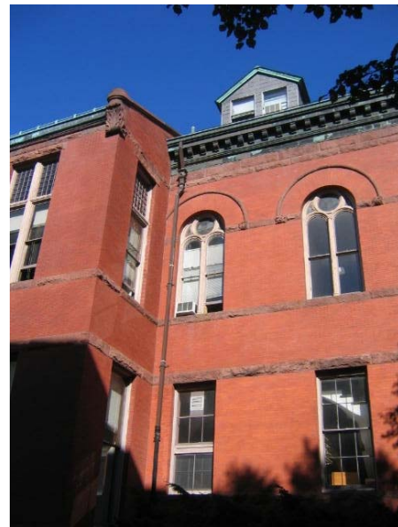
High & arched windows on the west side of the Superior Court Building
