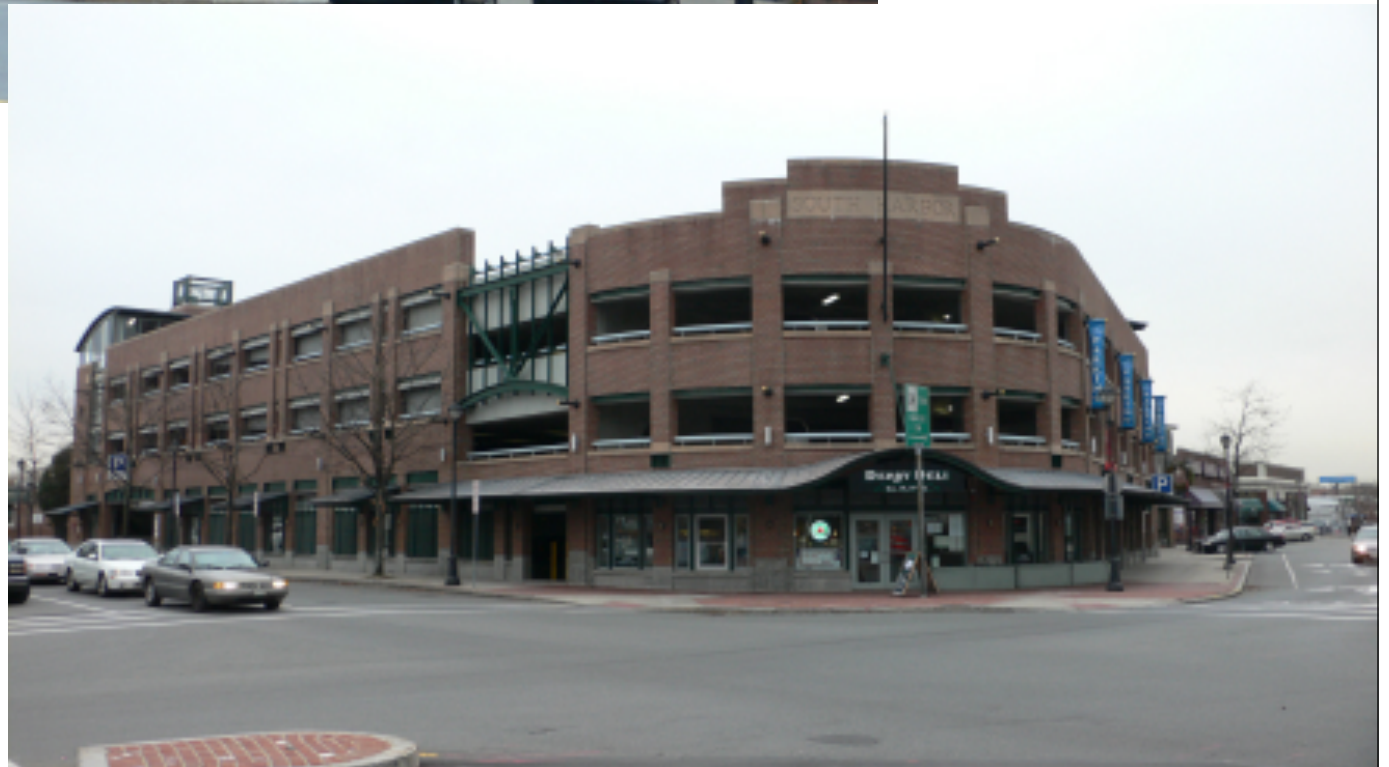
South Harbor Garage, Salem, MA
