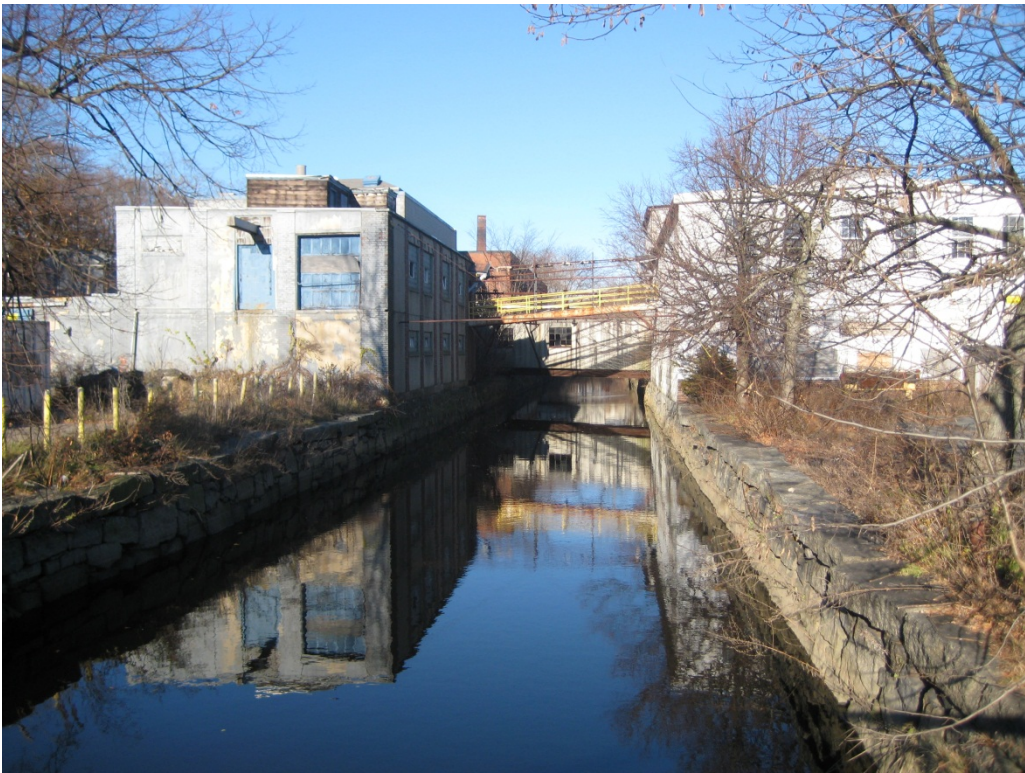
North River Canal Between 60 & 64 Grove Street. (Structure On the Left Side and Bridges Over Canal to be Removed)
