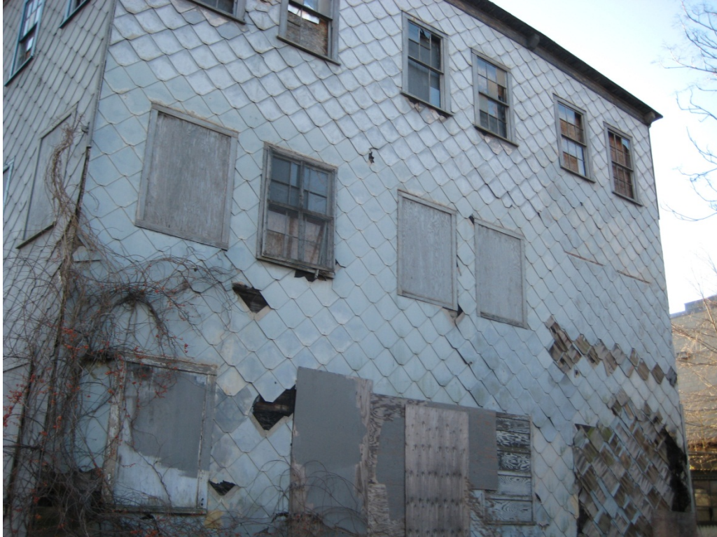
Rear of 60 Grove Street Office Building (To Be Renovated)
