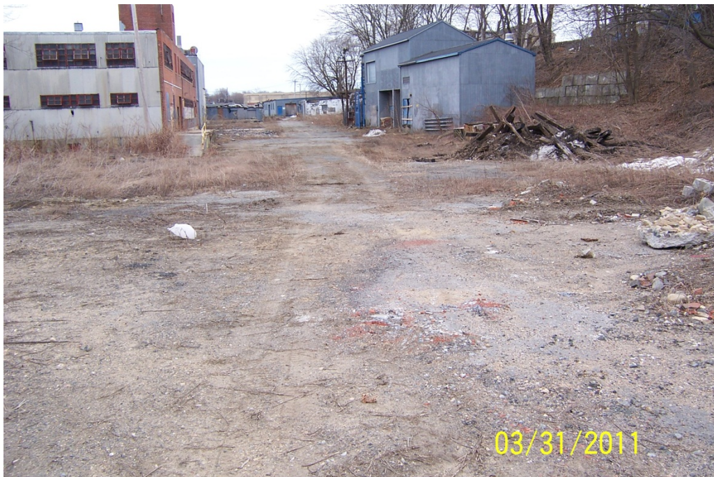
View From Rear of 64 Grove Street. Wastewater Treatment Building Located on the Right and Industrial Building Located on the Left. (To Be Removed)
