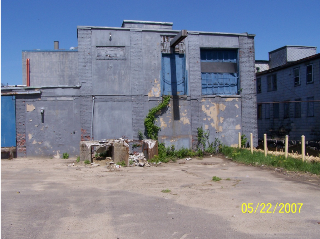
Front of 64 Grove Street Industrial Building (To Be Removed)
