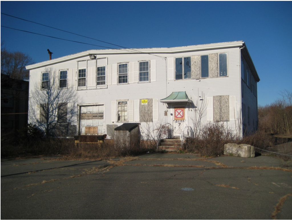
Front of 60 Grove Street Office Building (To Be Renovated)
