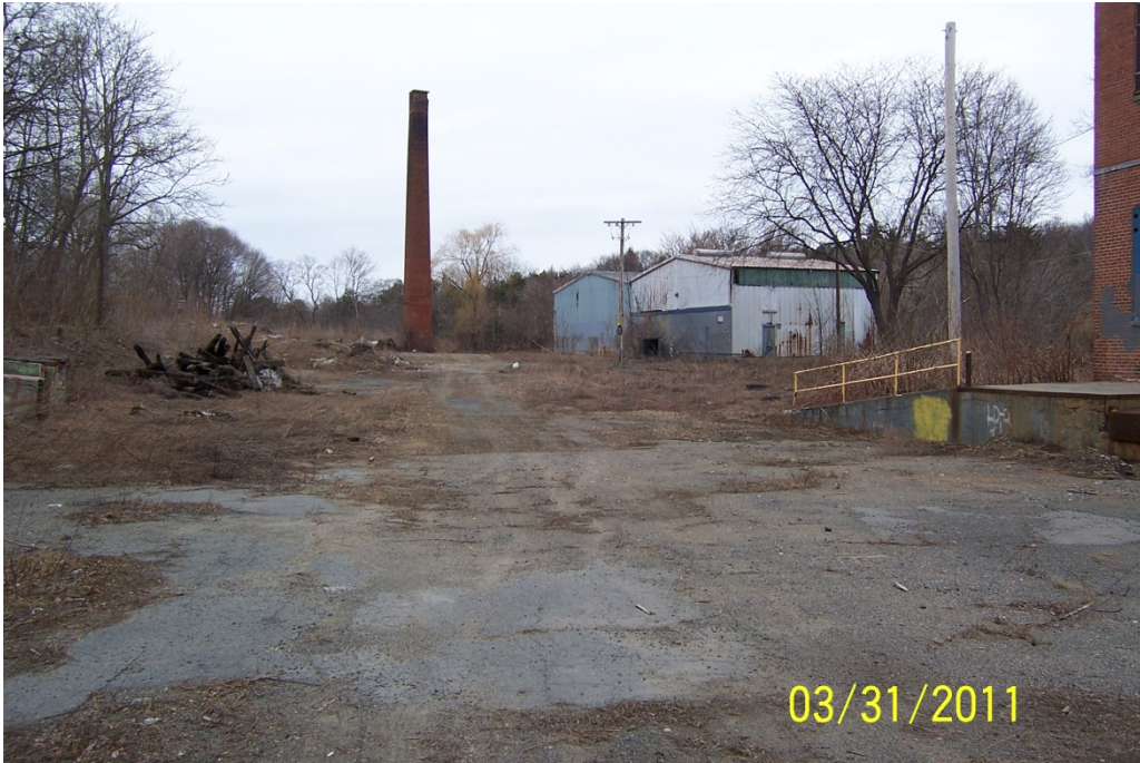
Rear of 64 Grove Street Property. Chimney From Former Sims Morocco Factory. (To Be Removed)
