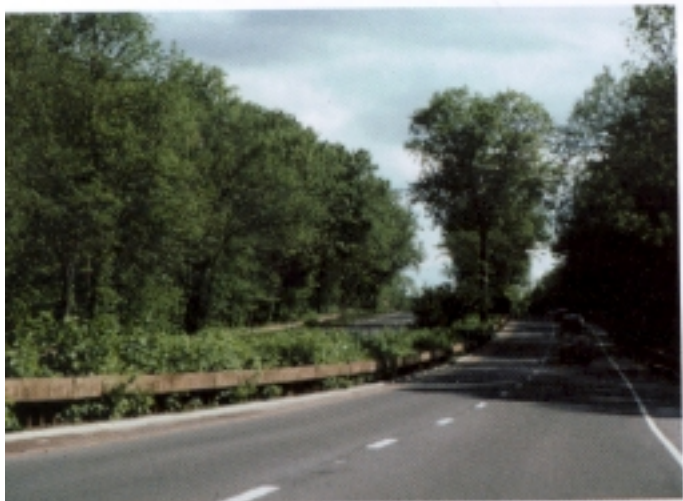
An advisory committee helped design a guardrail that was more appropriate to the parkway's historic context.
