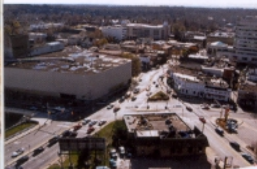
Before the roundabout was built, the gateway to Towson was dominated by cars waiting in long lines at traffic lights. Photo: Maryland State Highway Administration
